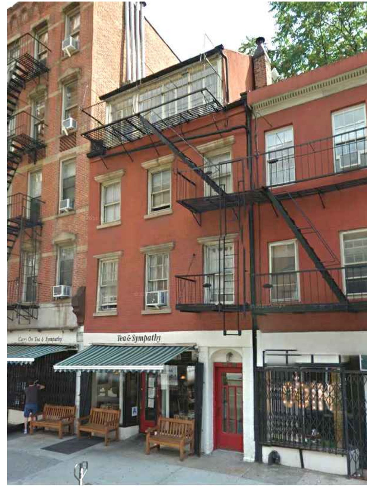
108 GREENWICH AVENUE, NY, NY
