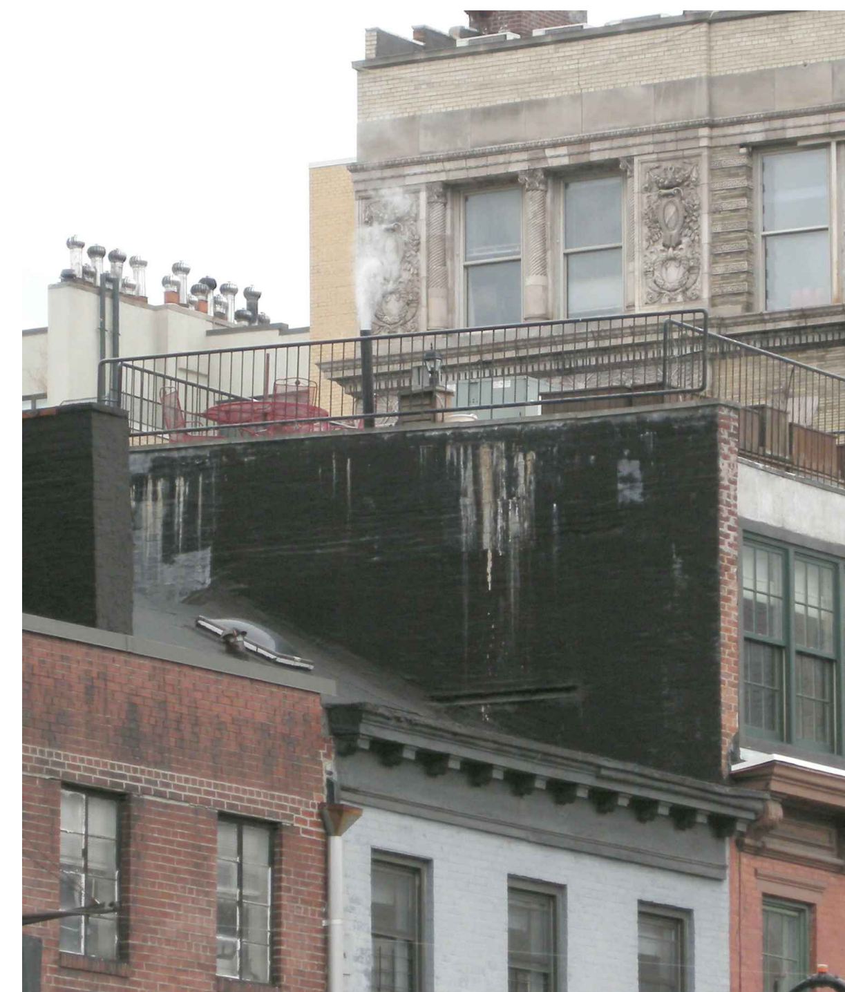
RP4 LOOKING AT AC UNIT FROM OPPOSITE CORNER OF 11TH STREET & 6TH AVE
