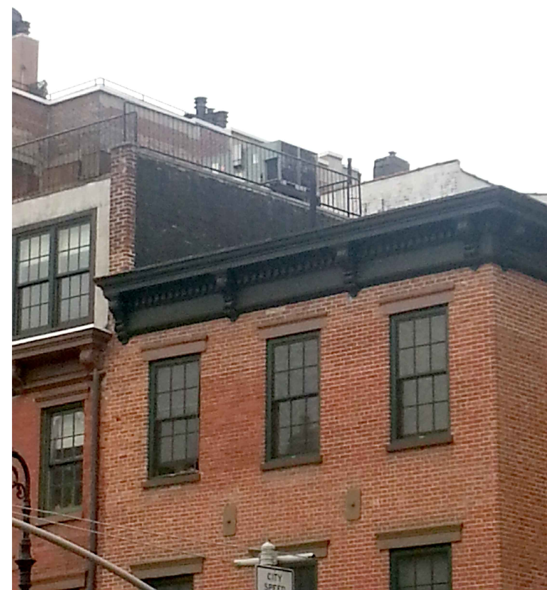
RP3 LOOKING AT AC UNIT FROM OPPOSITE CORNER OF 10TH STREET & 6TH AVE
