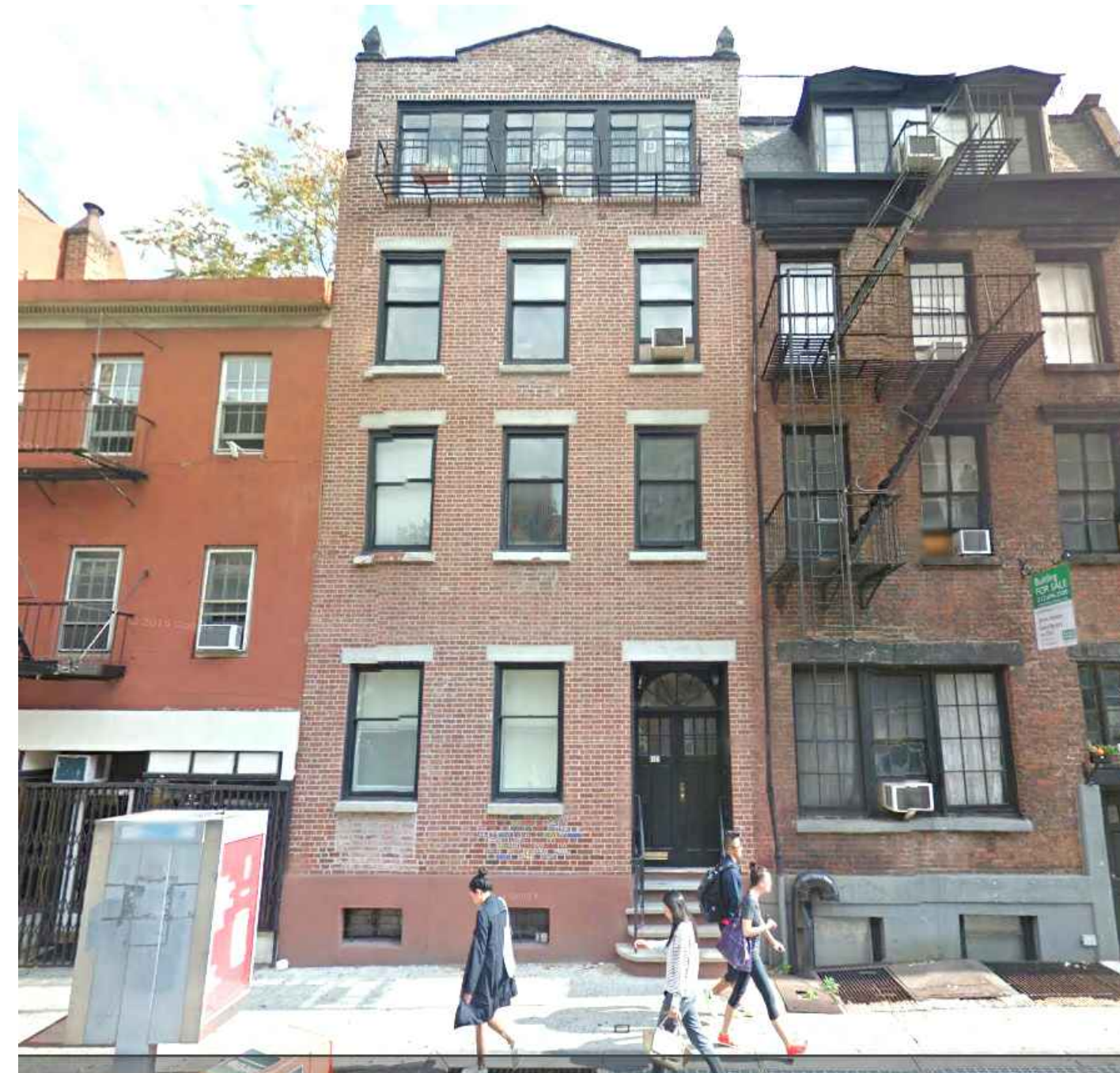
104 GREENWICH AVENUE, NY, NY
